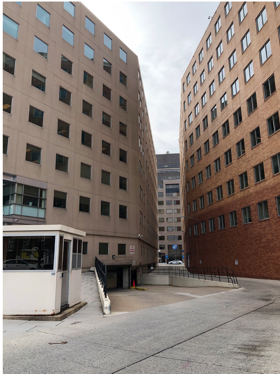
1. Public Alley, Looking South
