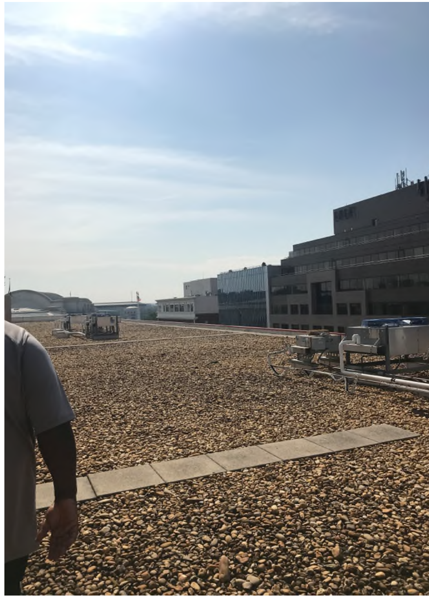
2. SE View from Roof
